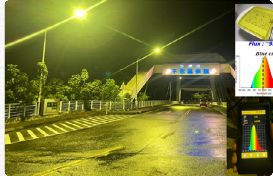
▲ Ecological Conservation Smart Lighting wave filter installed on streetlights in Kaohsiung Liuguei and spectrum of streetlights tested on site.
