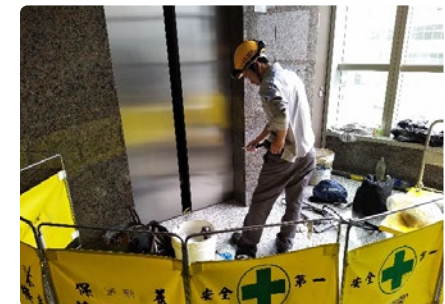
Contractor safety monitoring
