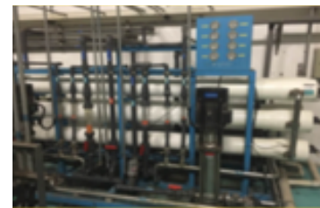
Reuse RO wastewater for cleaning toilets.
